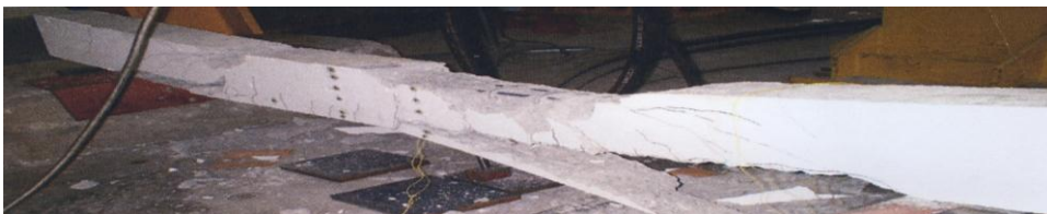
Fig. 8. Failure mode for strengthened beam without end anchorage C-F-0
