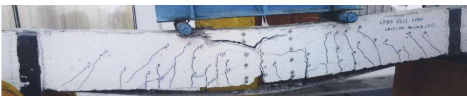
Fig. 9. Failure mode for strengthened beam with end anchorage C-F-75
