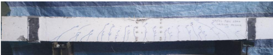
Fig. 7. Failure mode for strengthened beam with end anchorage S-F-85
