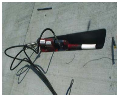
Fig.5. The monostrand stressing ram used from the central stressing pockets [10]
