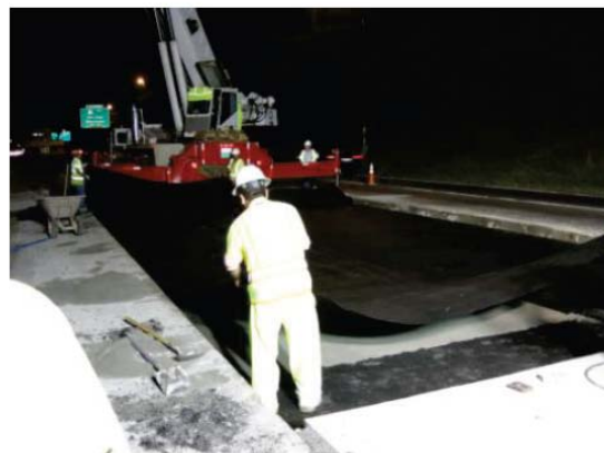
Fig. 14. Geotextile fabric is placed as a friction reduction layer [13]
