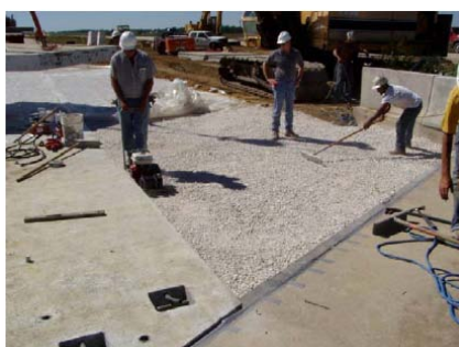
Fig. 12. Prepare the aggregate base [12]
