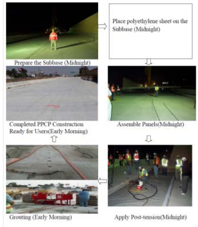
Fig. 3. The Construction Process of CaDOT's Demonstration Project [5]
