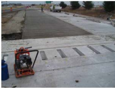
Fig. 8. The cast-in-place pavement constructed adjacent at the end of PPCP section [11]
