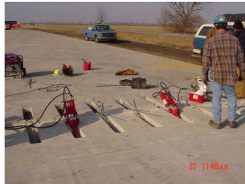
Fig. 10. Post-tensioning from the joint panels [11]
