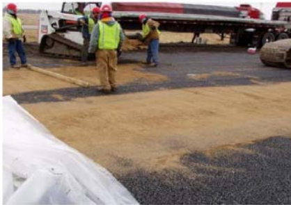
Fig. 9. Sand filled in the Permeable Asphalt Treated Base [11]
